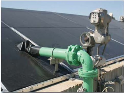
PIPE PENETRATION BOOT
