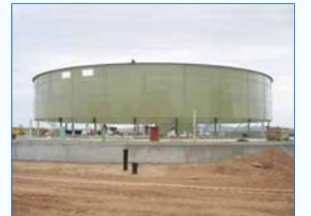
*Synchronized jacks are used to erect bolted-panel tanks from the ground up. Workers stay on the ground and perform no hot work which makes tank construction safer compared to field-welded methods.*
